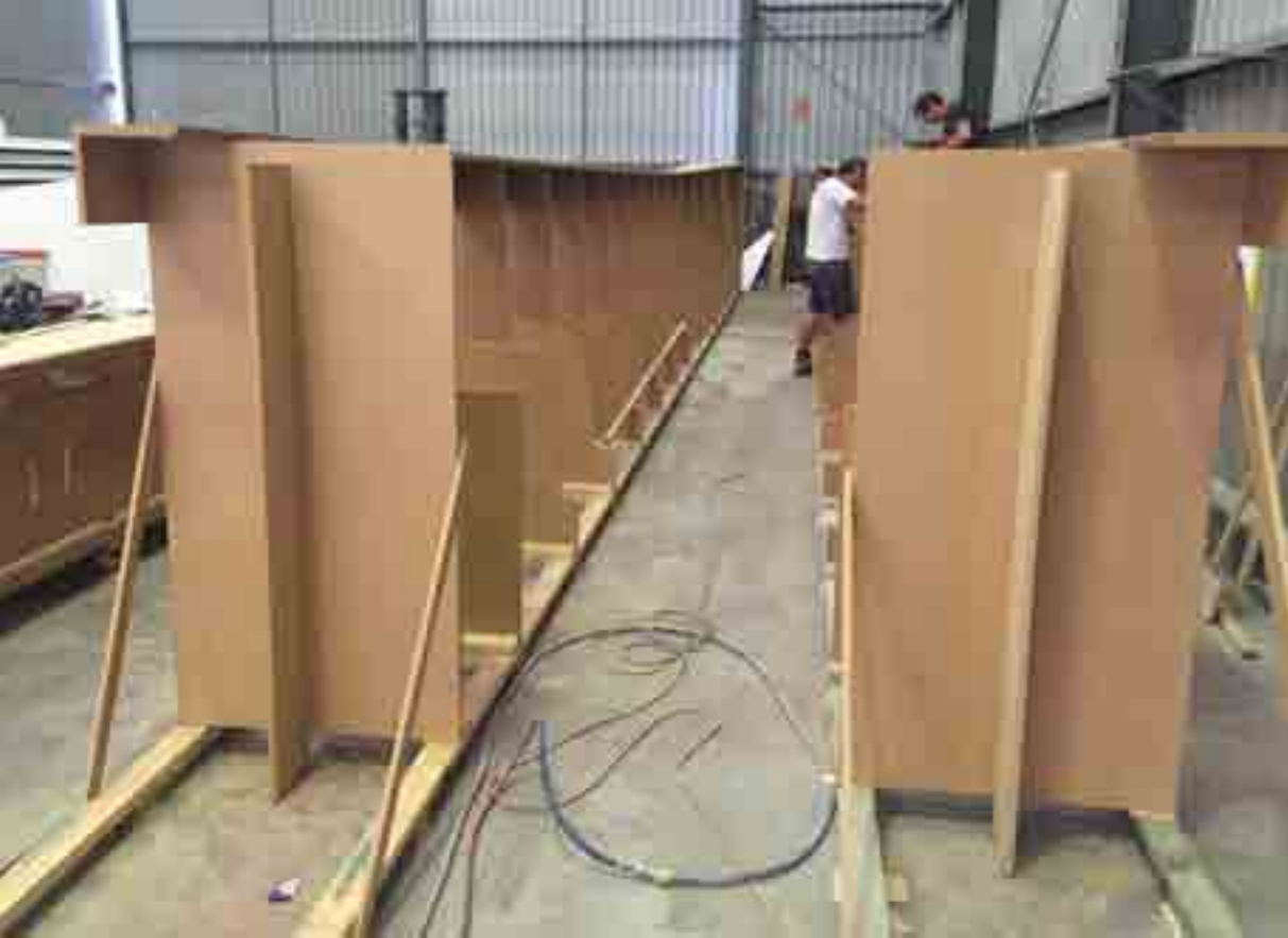
A new 52ft bottom will be moulded to further extend the Pathfinder M range.
